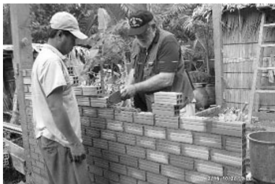
Laying bricks for new home in Giong Trom
