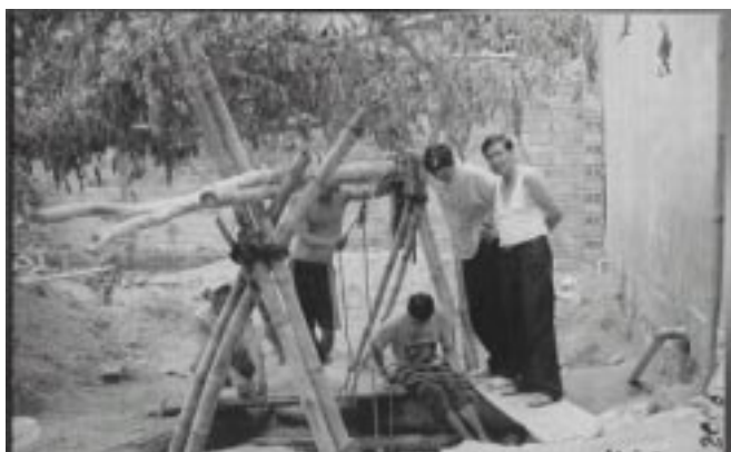
Water well under construction in Phu Yen province
